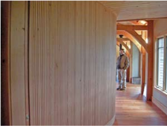
T&G Douglas fir with one-inch exposure adds corduroy texture to curved entry wall of master bedroom
